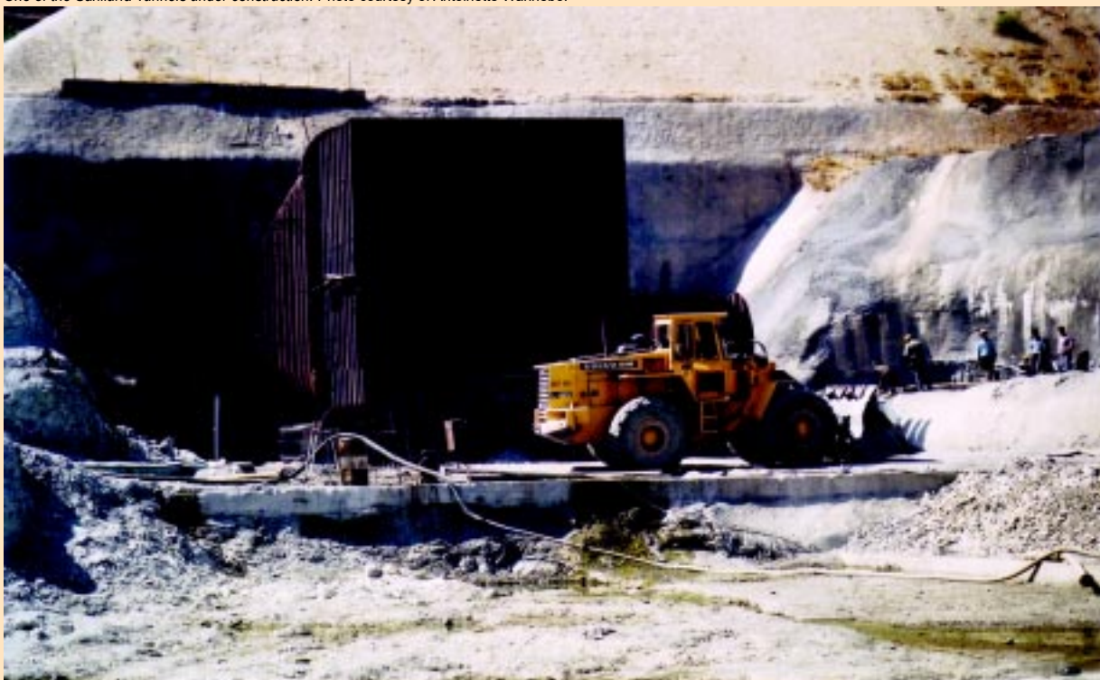
One of the Sanliurfa Tunnels under construction. Photo courtesy of Antoinette Wannebo.
