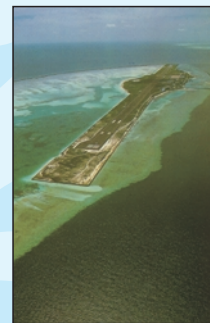
Maldives International Airport only 1.5 metres above sea level
